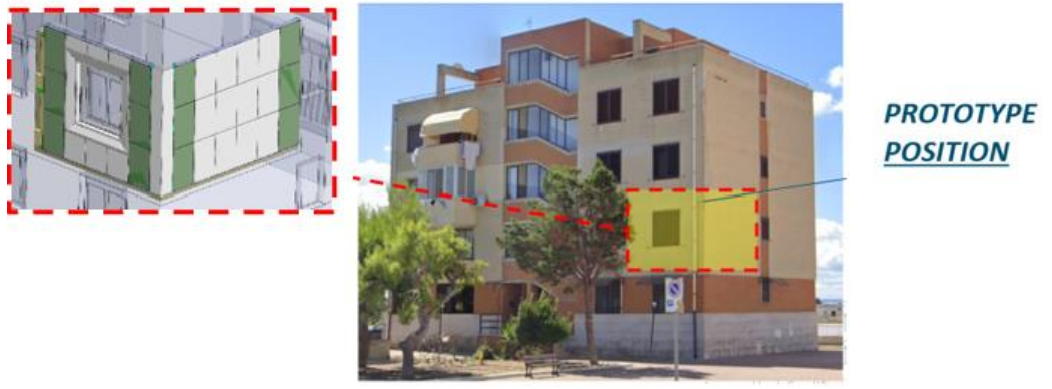
Figure 22: Prototype position on the Demo-site building
