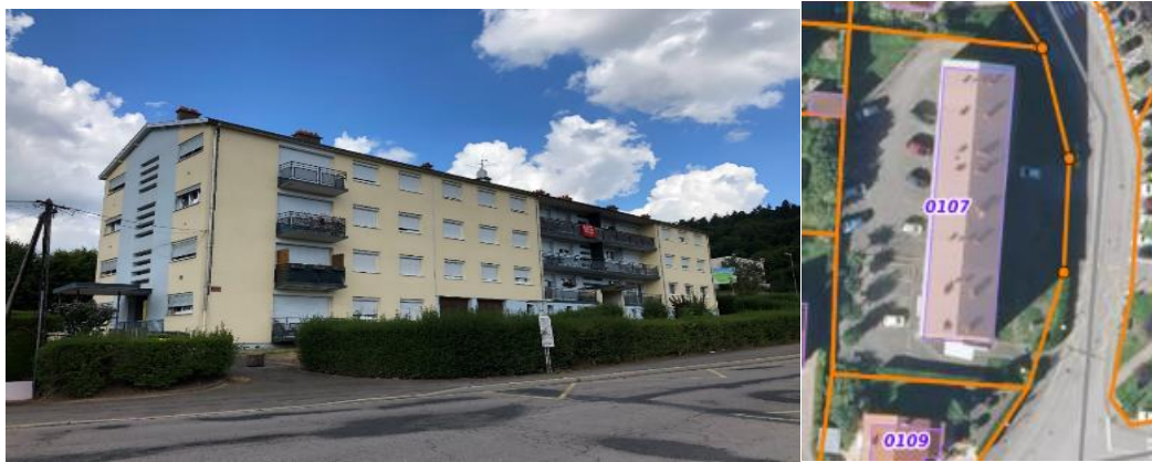
Figure 181. General view and aerial view of the French Demosite
