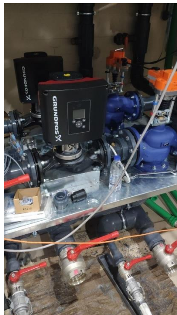
Figure 20: The pumping system of the testing facility
