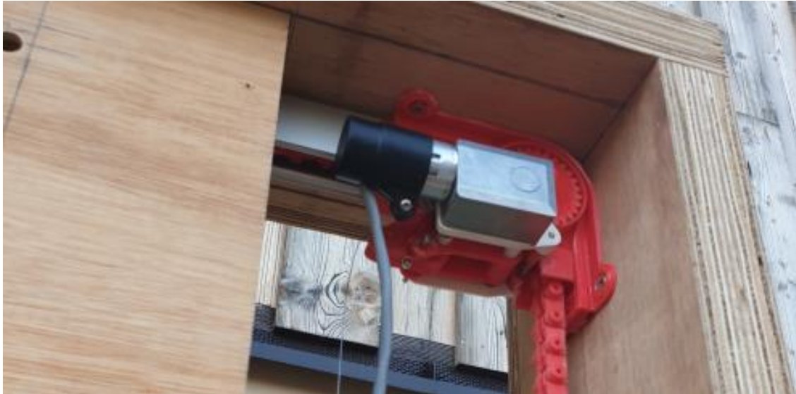
Figure 13: Intelligent Window System moving engine and moving parts
