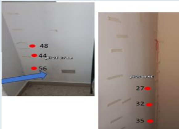
Figure 87: Wall and column thermo-hygrometric measurements
