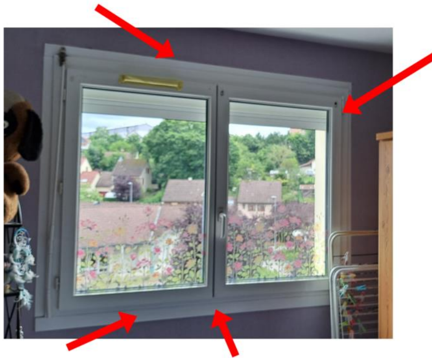
Figure 28: air inlet at wall frame connection.
