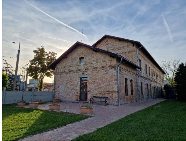
Figure 21: The Hungarian demo building - View from the courtyard, looking east.
