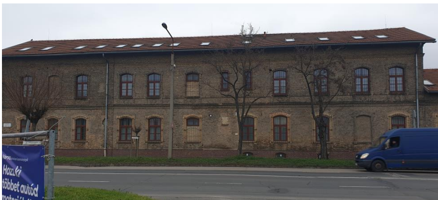
Figure 20: The Hungarian demo building - View from the street front, From south-southwest.
