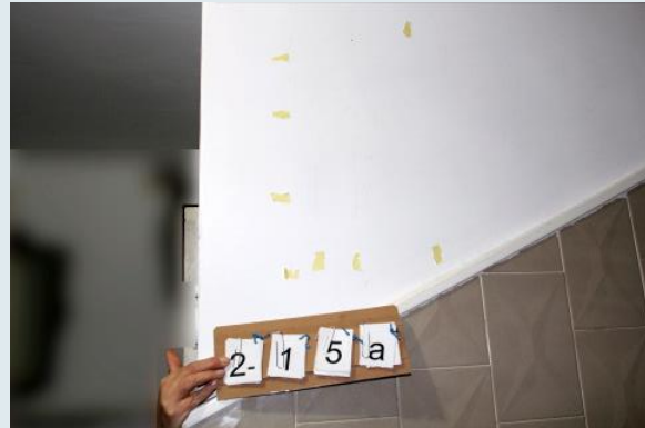
Figure 96: Labelling of reinforcement bars at column 15 on the second floor, stairwell side.
