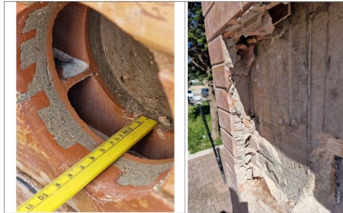
Figure 36: Results of the coring tests
