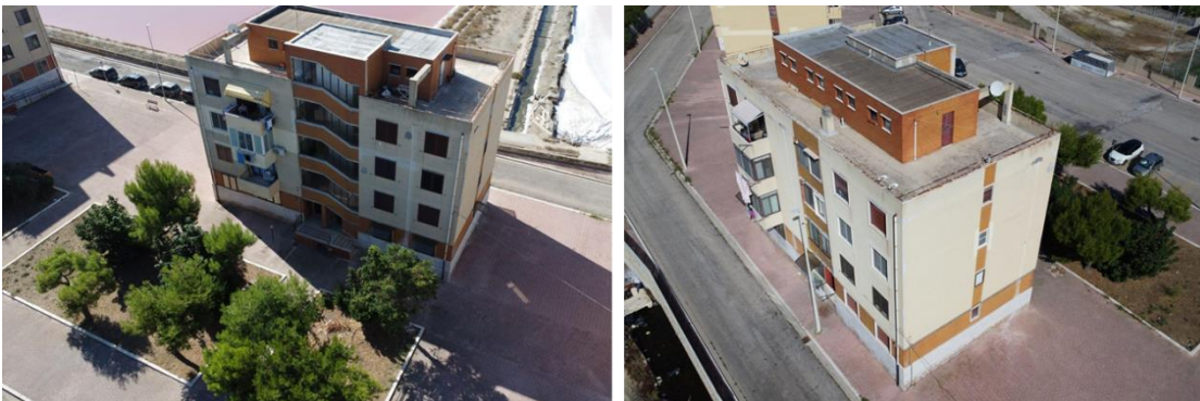
Figure 32: Picture of Italian Pilot Building
